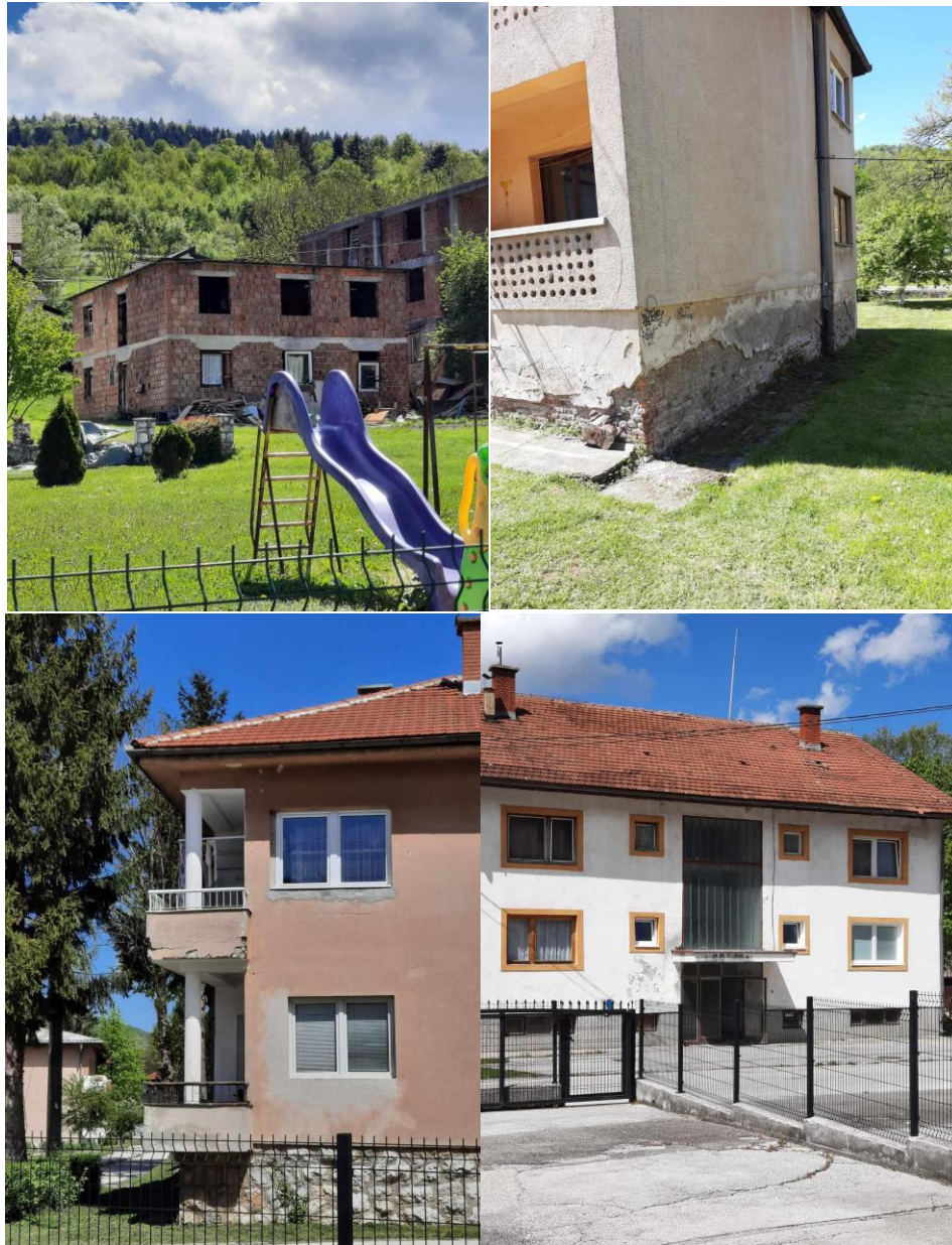
Figure 22 Building types identified by the survey in Hadzici
