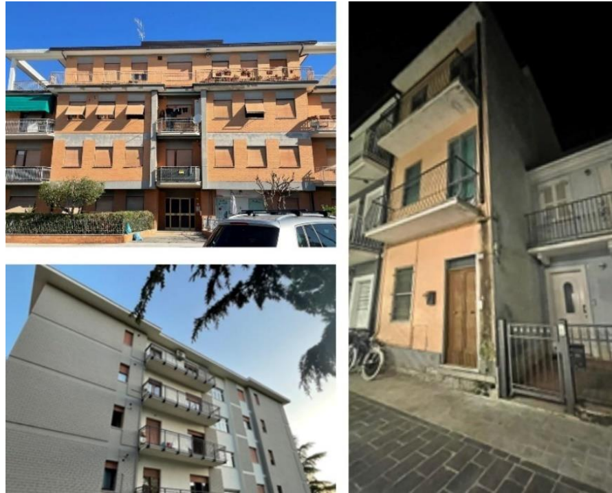
Figure 13 Left-up photo: Building in very good conditions, Left below: In good status, Right: Low quality
